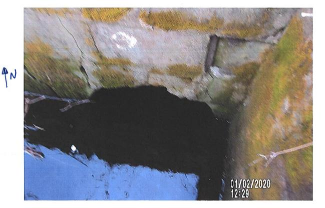
PICT # 2614 IS LOOKING NE AT 30" CMP OUTLET IN DRAINAGE STRUCTURE WITH WATER LEVEL AT 211/2" PILT # 2615 IS LOOKING NE AT OPEN DITCH FROM RR ALLESS DRIVE AND 30" CMP OUTLET. 75'S SW OF FENCELINE WEST
