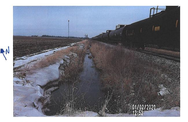
PILT#2627 IS LOOKING WE FROM RIC ALLESS 700'S NE OF FENCELINE WEST. 36" CMP OUTLET WATERLEVEL AT 18" WITH 7" MUCK IN FL.
