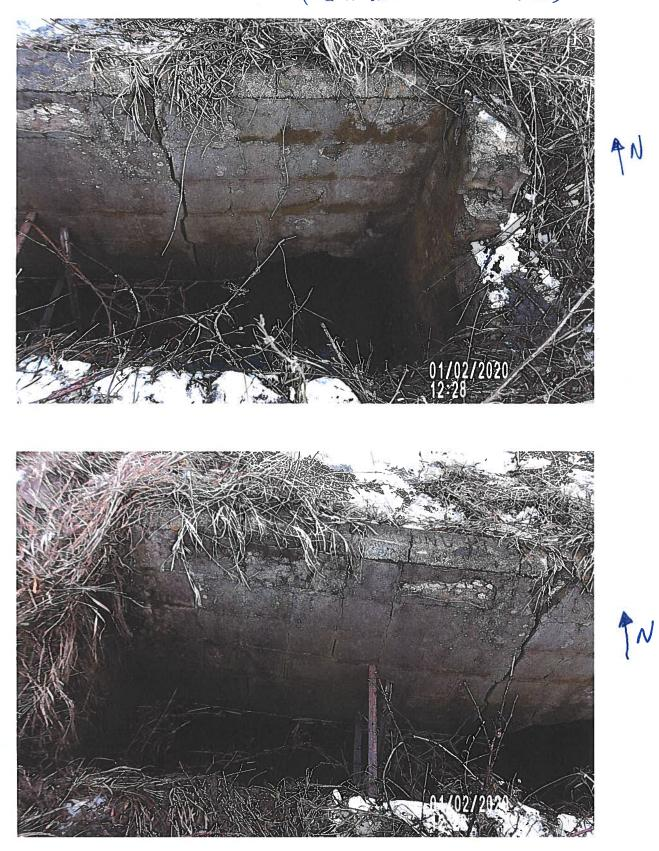
PILT#2612 IS LOOKING NEATDRAINAGE STRUCTURE (NW 1/2 OF STRUCTURE SHOWING IT IS IN POOR CONDITION, PILTHZELS IS LOOKING NO AT DRAINAGE STRUCTURE SHOWING IT IS IN POOR CONDITION
