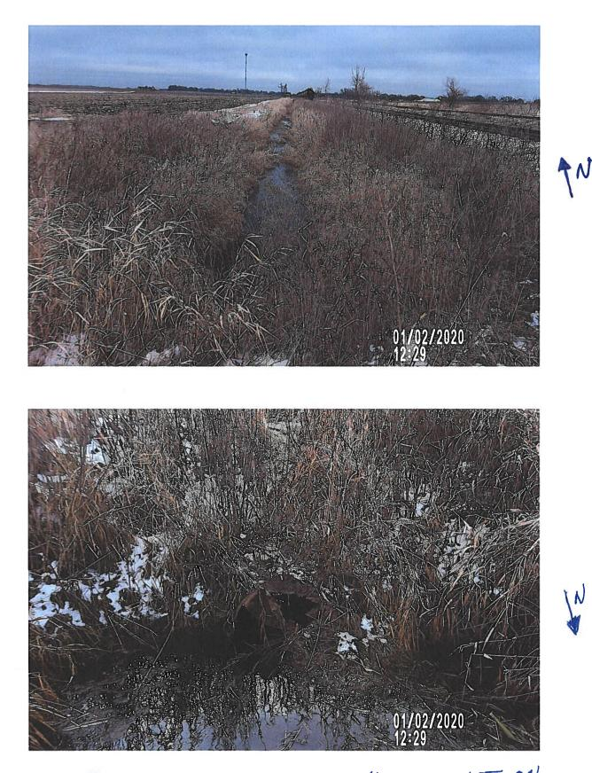
PICT # 2617 IS LOOKING SW SHOWING 30" CMP OUT LET ON NUSIDE OF RR ACKESS PRIVE ON NE SIDE OF DRAINAGE STRUCTURE WITH END CMP ALL MANCLED UP BUT FLOWING WATERLEVEL AT 20" PICT # 2618 IS LOOKING SW AT 15" EMPINLET (WATERLEVEL AT 11") IN SW CONER OF DRAINAGE STRUCTURE.
