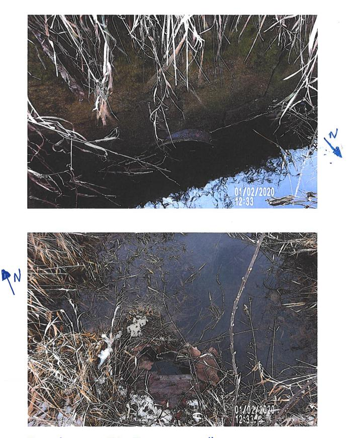
PICT# 2619 TOP VIEW OF MANGLED 30" CMP OUTLET ON NESIDE OF RRACCESS DRIVE PICT# 2620 is LOOKING WEST AT DRAINAGE WEIR JUST SOUTH OF FENCELINE WEST SW CORNER OF WEIR IS A 6" CLAY PIPE OUTLET 1/2" FLOW
