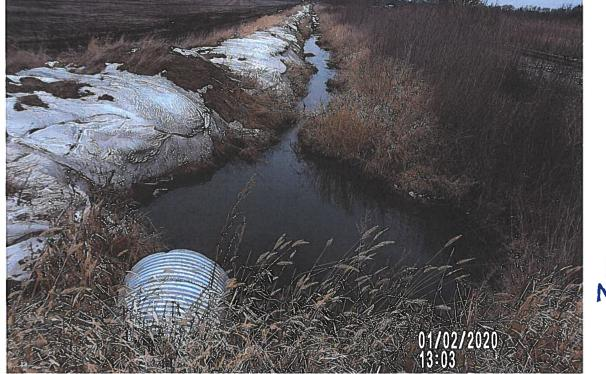
PICT # 2629 IS LOOKING NE WEST OF RRTRACKS & NORTH OF IOTH AVE (IIOTH STREET) SHOWING 48" CMP OUTLET O.15' ABOVE WATERLEVEL & 36" CMP OUTLET WITH WATER LEVEL AT 17" WITH 5" MUCK IN FLOWLING
